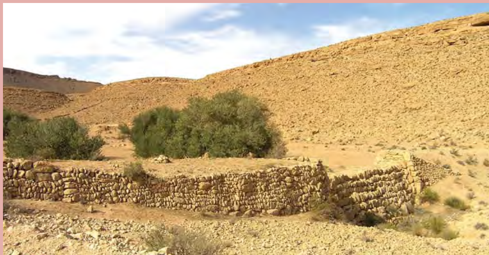
Traditional terracing to harvest water and control overland flow near Tataouine in Southern Tunisia.
